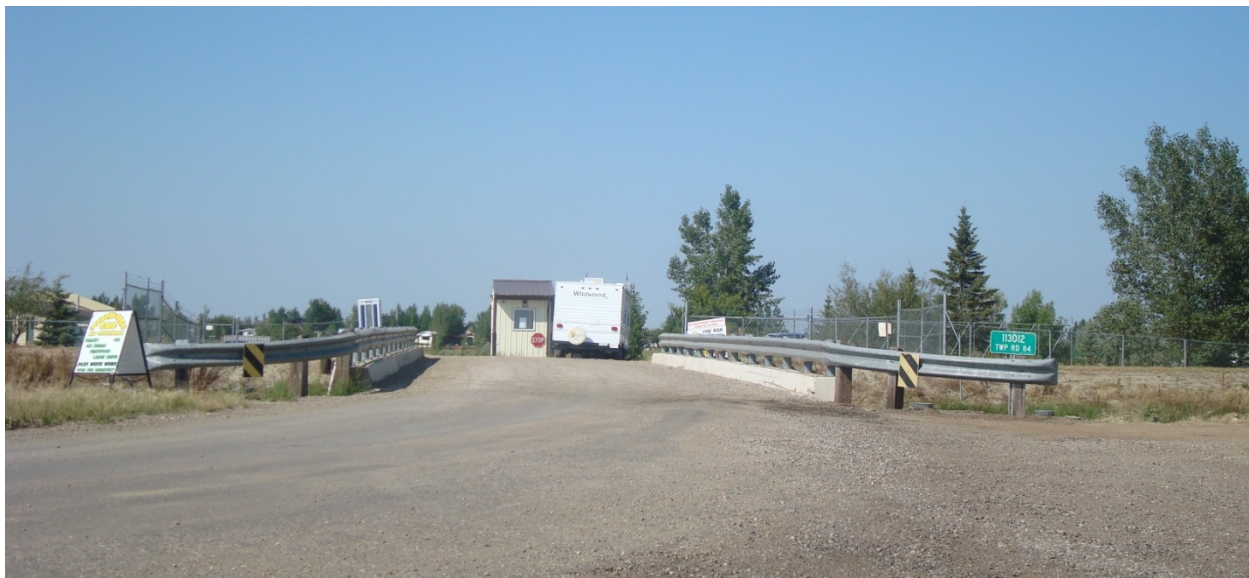
Existing Park Gate bridge and kiosk
