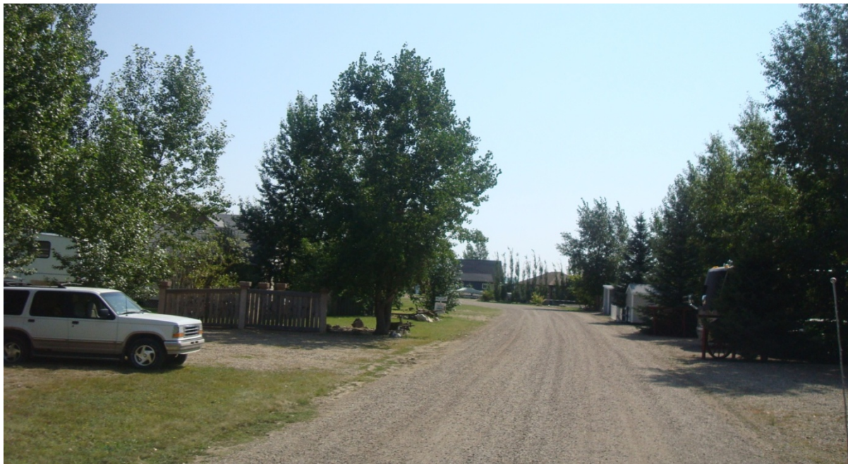
Existing local road on the Northshore
