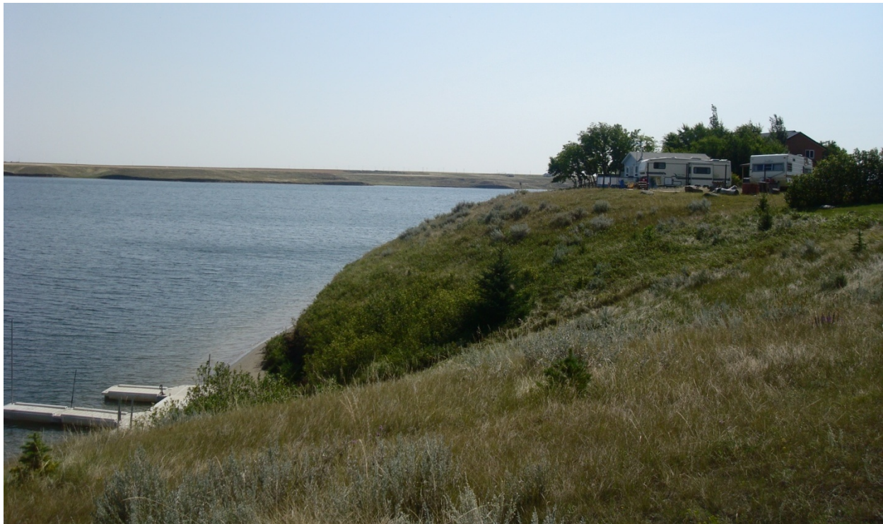
Northern shoreline showing area with potential slope instability
